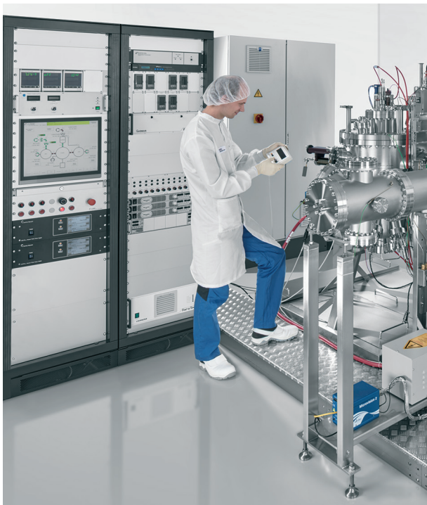
System control rack
